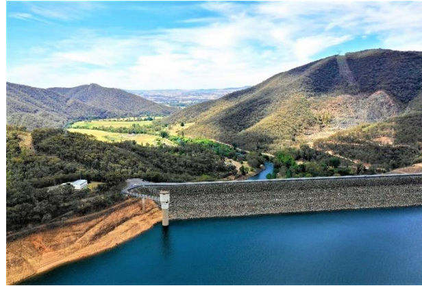
Blowering Dam wall
